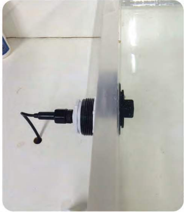
Probe installed! Now remove the 2" plug allowing water to be in contact with the Probe
