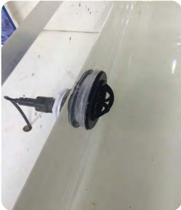
Install grate into wall fitting. Installation is complete, Continue filling you spa with water
